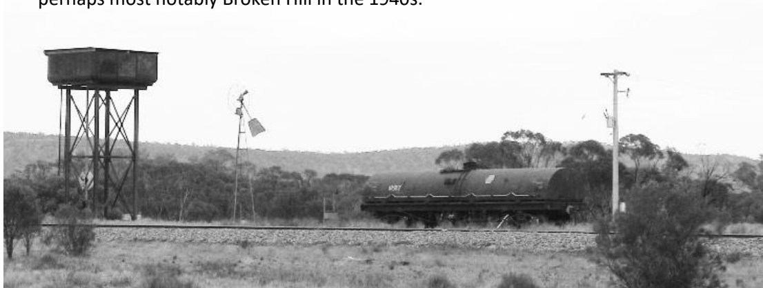
A bogie water tank standing at Roto in western New South Wales. Photo: I.W. Gray
